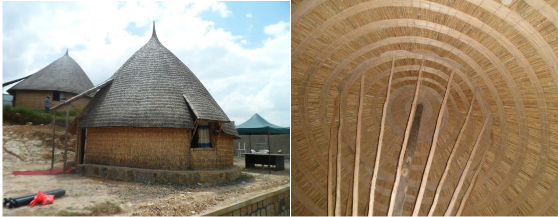
Figure 4.8: Improved traditional house (bamboo 'gojo' and a ceiling made from bamboo & wood beam)
