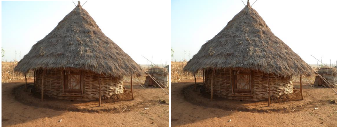
Figure 4.7: A circular Bertha Tukul made from bamboo, hardwood and dryland grass. The tukul is vulnerable to termite attack and have the shortest durability of all house types.
