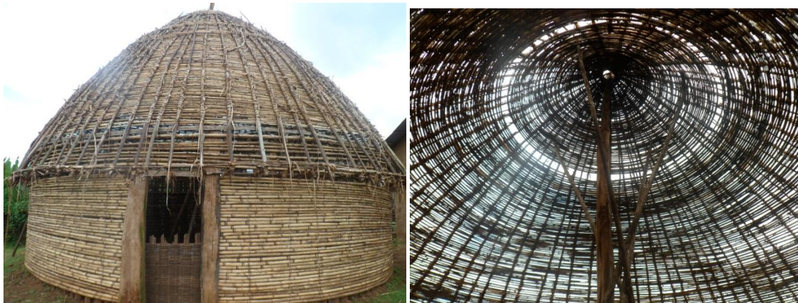
Figure 4.6: a typical traditional Gurage/Silie Houses where roofs and walls are made mainly from bamboo.
